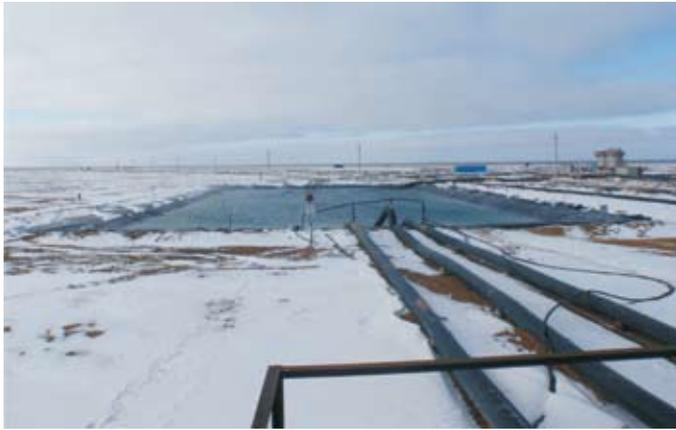
As confirmed by long-term studies, currently, uranium production using uranium drillhole in-situ leaching is the most attractive method of the uranium production in terms of process operations simplification. In this case, the Kazakh enterprises have excellent experience in application of sulphuric-acid uranium leaching in the territory of the South Kazakhstan Oblast. One of them is APPAK LLP, the first joint Kazakh-Japanese venture expanding to the industrial uranium production.
